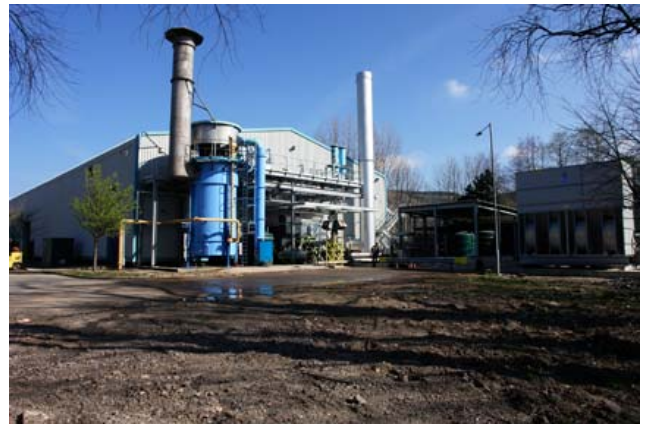
April 2007: Completed Facility Reconstruction at ECM2 – Port Talbot
