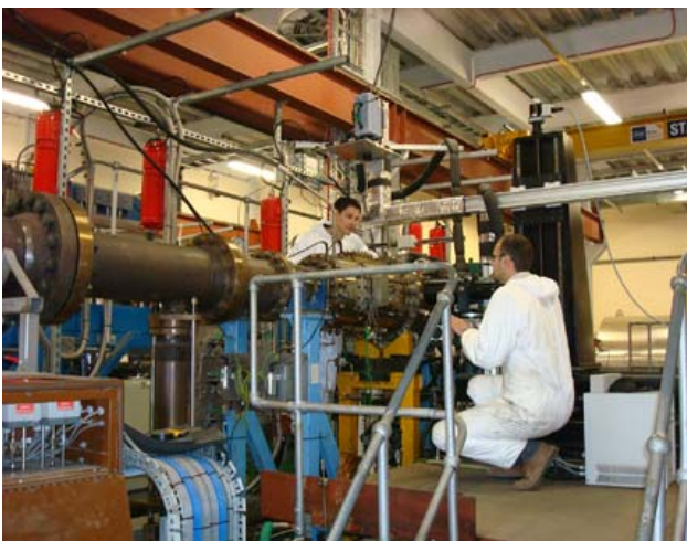
Commissioning the new optical combustion measurement section
